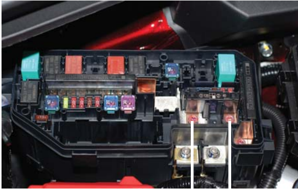
120 Main Fuse Screws
